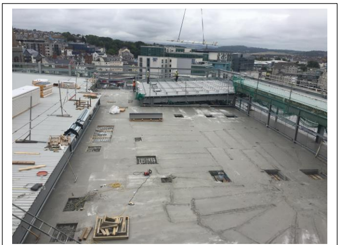
Concrete slab poured to the plant deck, roofing works ongoing.
