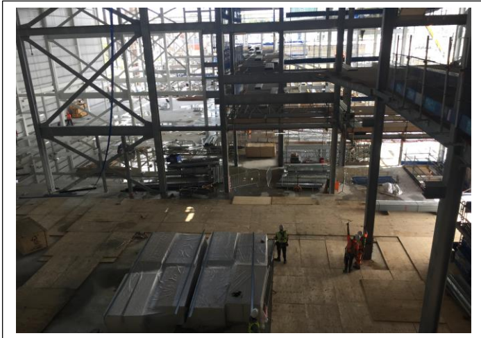
IMAX auditorium loaded out ready for dry lining.
