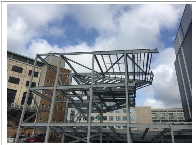
Steelwork installation ongoing to Zone 4.
