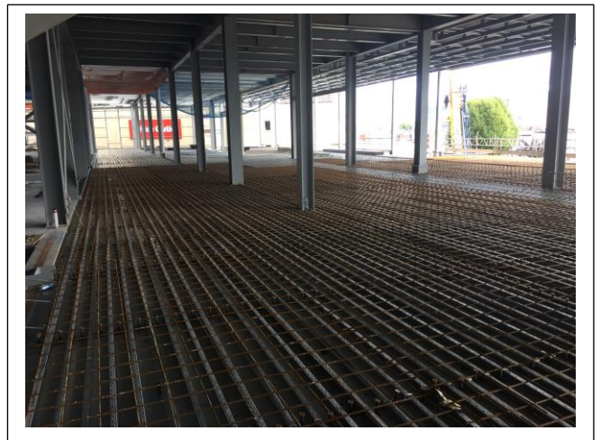
Preparation work ongoing to podium level, ready for concrete pour.
