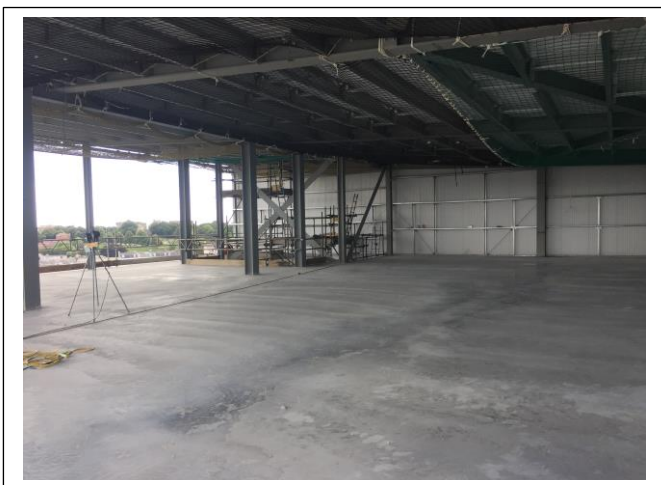
Concrete slab poured to the Sky Bar.
