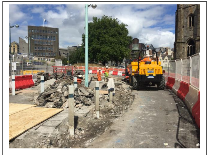
S278 works commenced to Charles Cross roundabout.
